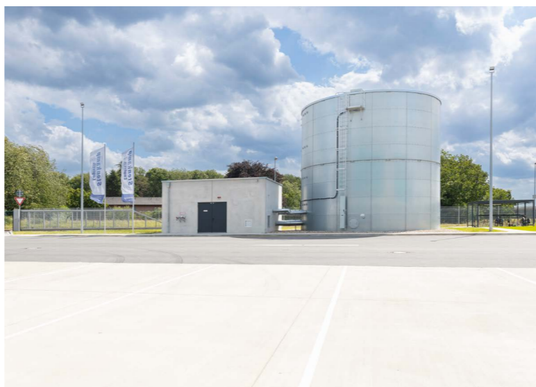
Innovative storage technology to buffer PV-generated electricity
