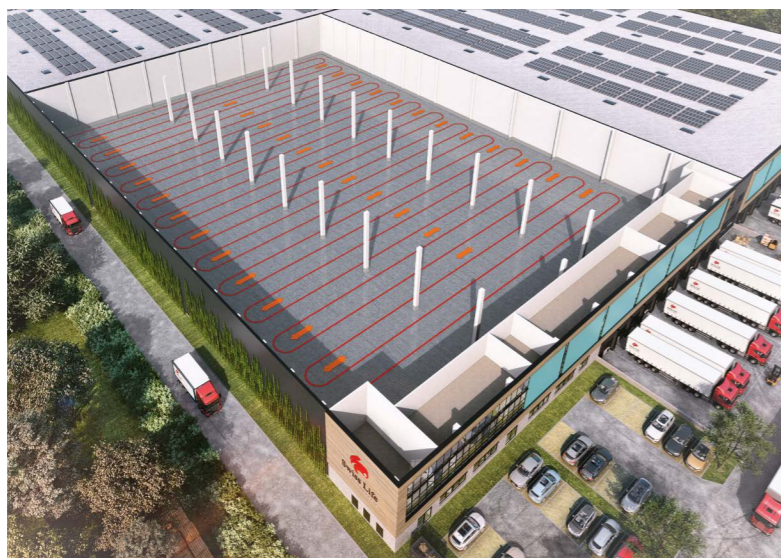
Heating and cooling loops built into the warehouse floor
